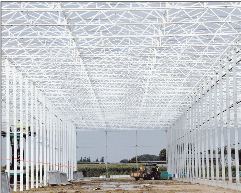
Construction is underway on a greenhouse facility that will produce locally grown lettuce along the frontage road of Interstate 35 just south of Richie Brothers Auctioneering by Medford. The greenhouse is expected to be completed by November with the first seeding taking place in late November. Revol Greens will be supplying lettuce before the end of the year to grocers and restaurants in a 200-mile radius around the Midwest.
