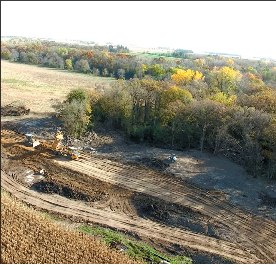
A crew builds a ravine-stabilization berm this fall on Dwane Hull’s property in Austin Township near the Cedar River.
