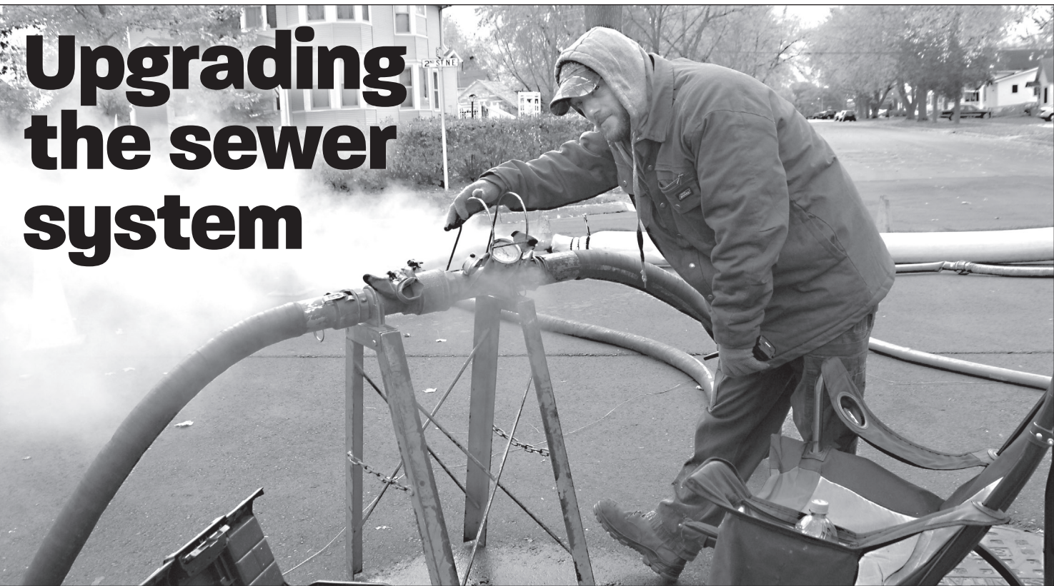
Workers installed new sewer system linings on the north part of Blooming Prairie last week. Joe Foster of Municipal Pipe Tool Co. of Hudson, Iowa, checks out a pressure meter while installing the linings.
