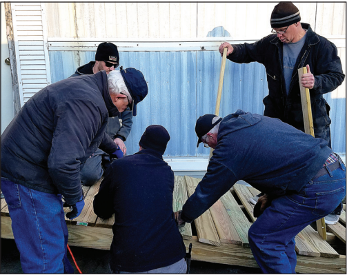
SUBMITTED PHOTO Volunteers from the Owatonna Church of Christ assisted the Steele County Beyond the Yellow Ribbon organization in replacing a ramp that was in disrepair for a Steele County Air Force veteran.
