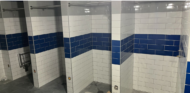
Locker Room Showers
