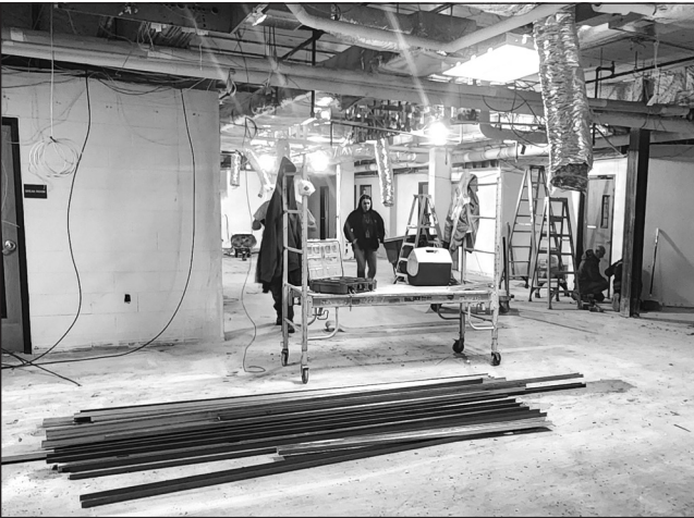
Work has begun on the new Rice Steele 911 Center. The 26-year-old consolidated dispatch center will move from Owatonna to Faribault later this year and will feature all new equipment and technology.
