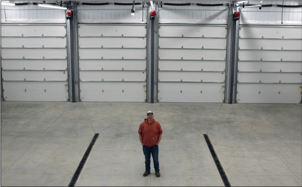
Fire Chief Logan Busho shows off the nearly completed fire hall, which will be fully functional and operational soon. The city plans to have an open house later this summer.
