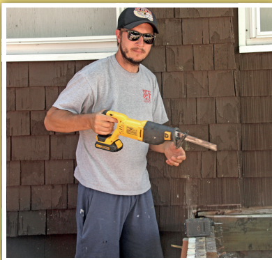
Brandon Guse uses a power tool to put together a new steps on the fairgrounds.
