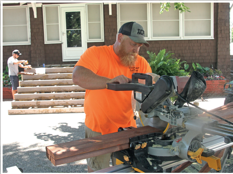
Scott Seykora of Owatonna operates a power saw while working on a repair project at the Mother's Rest building on the Steele County Fairgrounds. Brandon Guse is shown at the steps in the background. The two are art teachers who work at the fair during the summer.
