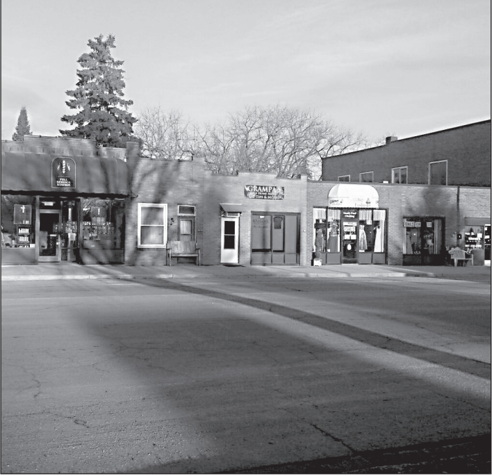
Medford's Main Street was the initial location of the fire hall and city offices back in 1937. Medford city officials are pushing state lawmakers for financing to help build a new Medford Municipal Complex. "We need this," city officials say.
