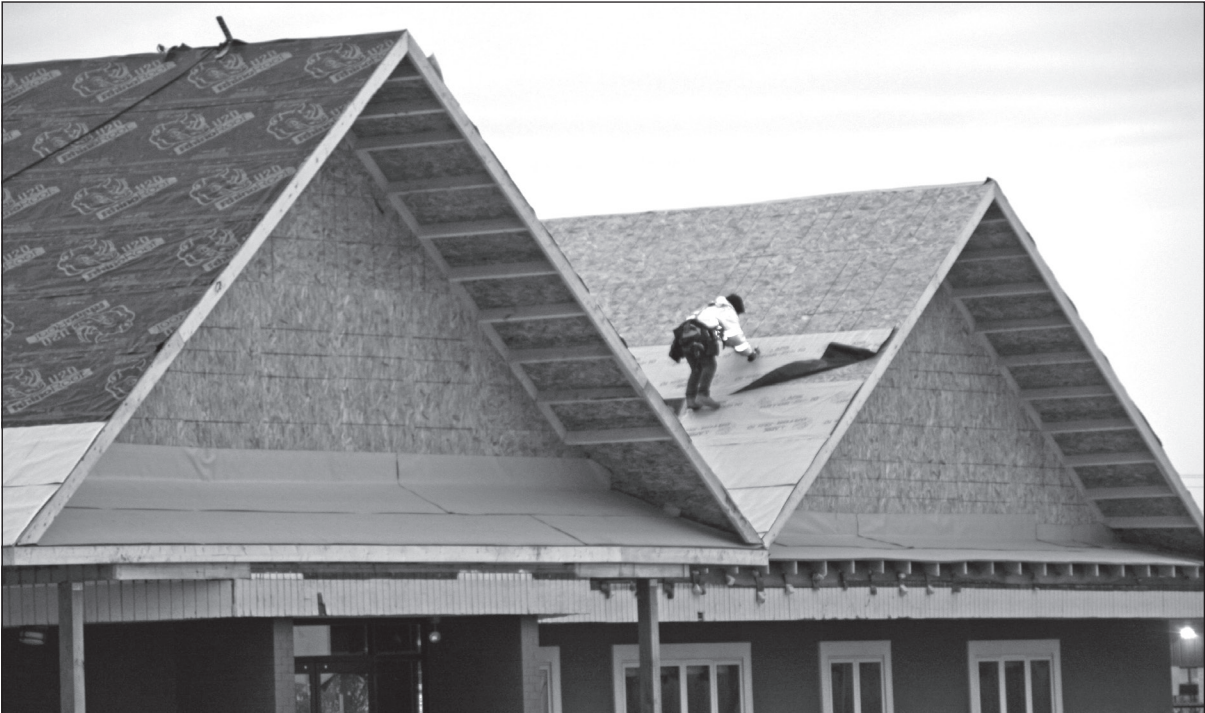
A construction crew works late last week on the new pitched roof of the Leo Augusta Children's Academy in Blooming Prairie. The former Minimizer building is being remodeled, and will include more than 18,000 square feet of building and land renovations on three acres. The facility will "deliver a hands-on model of child development," its website says, with the capacity to serve more than 100 children, infant through age 12. It's scheduled to open this spring.
