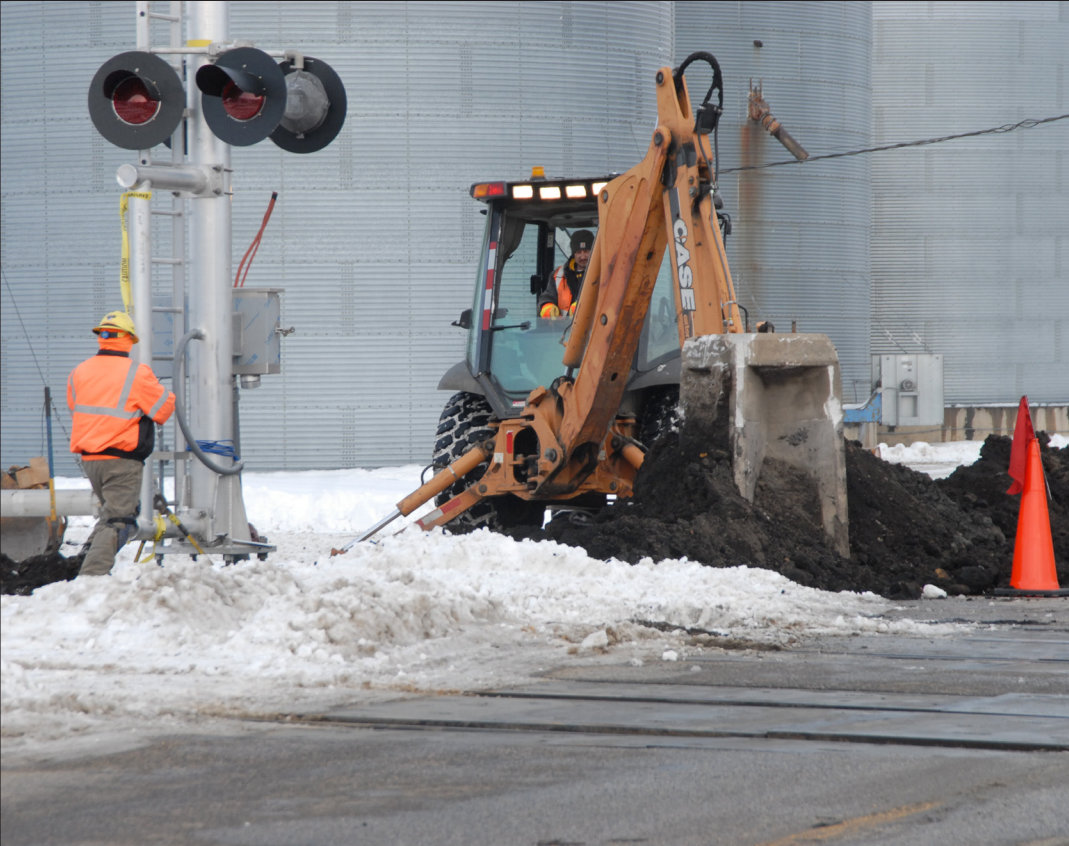
Workmen for the Union Pacific Railroad have been busy recently updating the railroad signals in downtown Ellendale on Highway 30. New signal arms have been installed.
