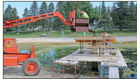
STAFF PHOTO BY HOWARD LESTRUD More concrete is brought from the northwest part of the Pine Springs Pool to be placed on the table of the diving platform. The platform is elevated 9 feet.
