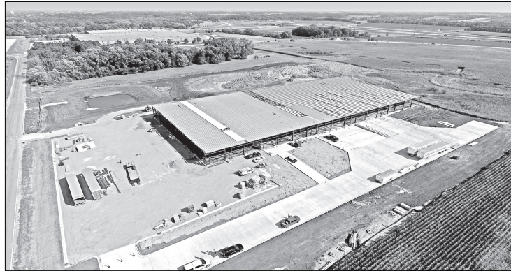
This is what the new Minimizer plant looks like as construction progresses at its new location in Owatonna. Minimizer hopes to move its entire operation from Blooming Prairie to Owatonna by February of 2021.
