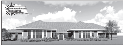
This is a rendering of what the new Southeast Regional Crisis Center will look like. It's currently under construction in Rochester and will serve all of southeast Minnesota, including Steele, Dodge, Waseca and Mower counties.
