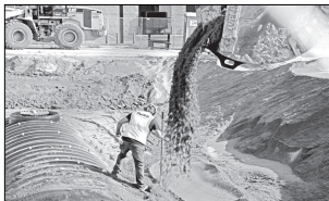
Workers fill a hole with sand to make room for a new on-site fuel station at Cashwise Foods in Owatonna. The station is being constructed in front of the current store. Shoppers will soon not only be able to purchase groceries and liquor at Cashwise, but also fuel. Construction should be completed later this fall.
