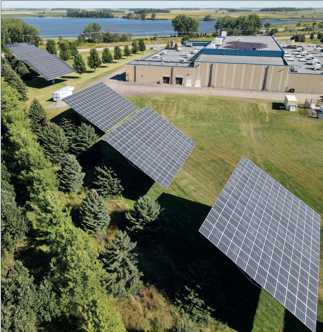
A solar tracker is on the grounds of Lakeview High School in Cottonwood, Minn. Mark Oeltjenbruns of Claremont is looking to install more of the systems with his new company, Agrisun Energy and Repair.
