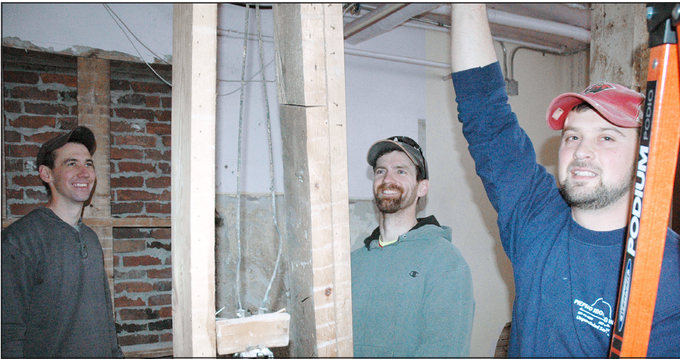
Staff photo by Howard Lestrud Weinberg Construction, LLC of Owatonna is doing some major remodeling of bathrooms at the First Baptist Church of Blooming Prairie. Work crew members include brothers James Piepho and Curt Piepho and Phil DeMarte.
