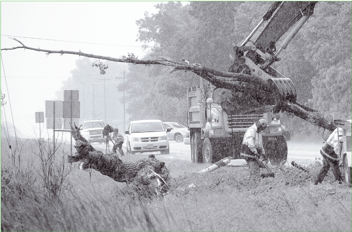
Staff photo by Rick Bussler Highway crews responded to the area of County Road 14 at SW 128th Street to remove a large tree from the roadway during a severe thunderstorm that rocked Steele County on June 17.
