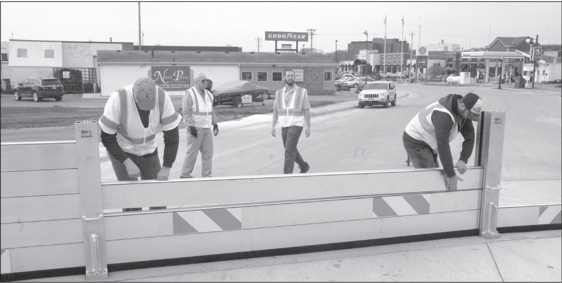
Staff photo by Howard Lestrud Workers install a removable flood wall on a street in Austin near the Cedar River. The aluminum flood wall was purchased by the city to prevent major flooding in the future.
