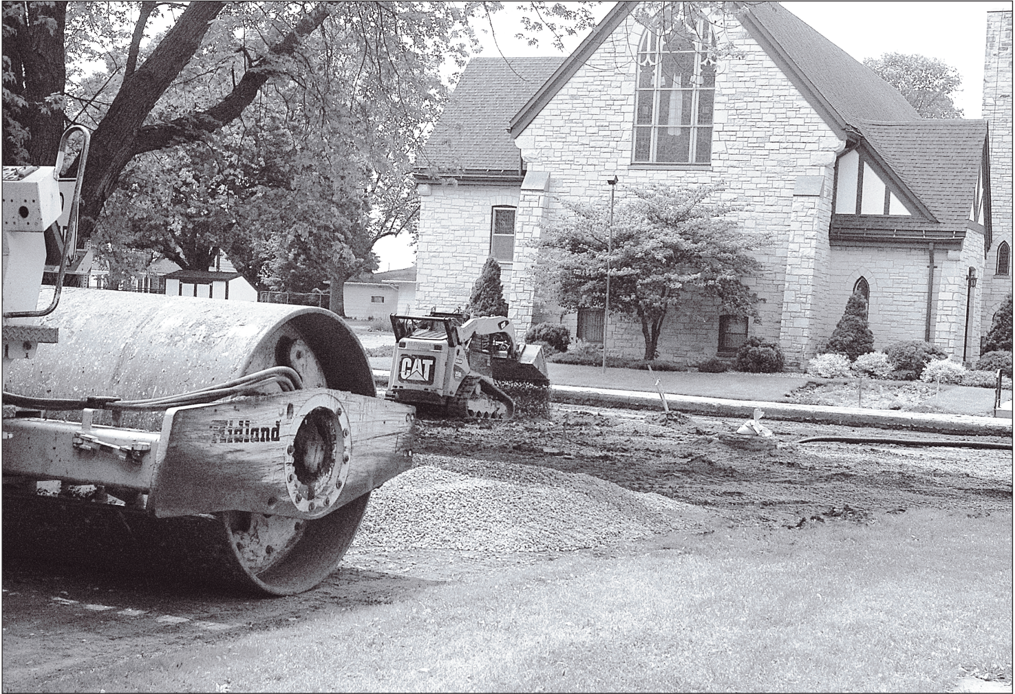
Construction season is in high gear in the city of Ellendale as workers reconstruct 4th Street as it intersects with 5th Ave. The street being reconstructed passes by First Lutheran Church.
