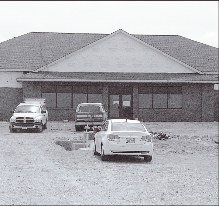
Staff photos by Howard Lestrud Casey’s General Store will have a new store open shortly in Ellendale. Construction continues at a rapid pace.
