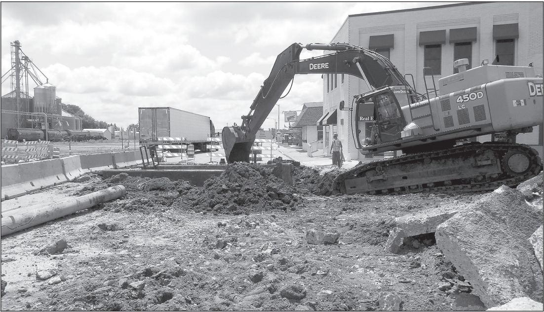
Staff photo by Howard Lestrud Elcor Construction of Rochester has been busy working on water main and sanitary sewer reconstruction on Main Street in Blooming Prairie. All kinds of traffic continue uninterrupted on Highway 218 (note semi-truck going south). The $2.7 million project began on June 15 and is expected to be completed by Nov. 1.
