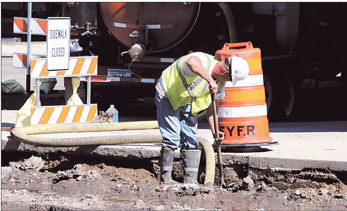
Staff photo by Jake Nelson Construction work continues on Main Street in Blooming Prairie. Above, workers continue their efforts on Main Street, despite some recent rains, which resulted in a soggy surface to work with.
