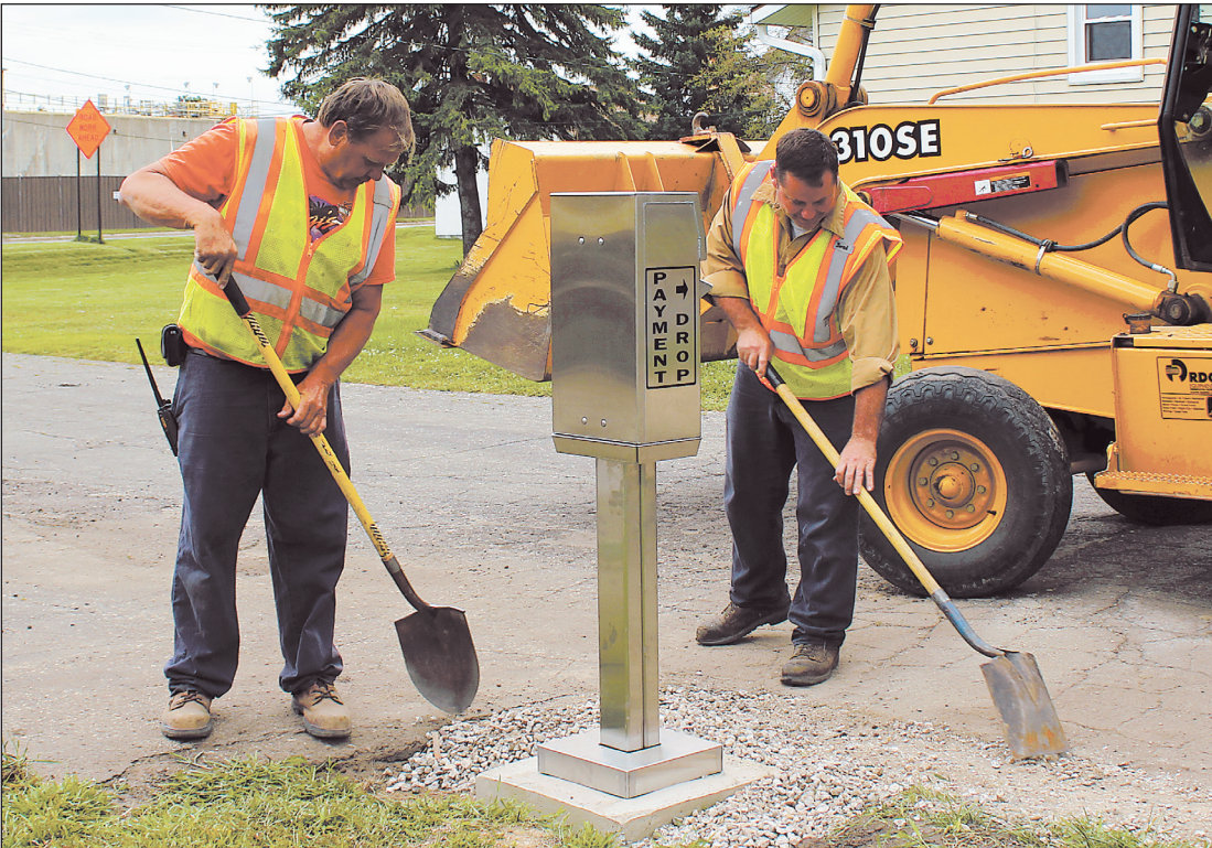
Staff photo by Laura Berndt Tom Swenson and Jared Brown are hard at work installing the Blooming Prairie Public Utilities' payment dropbox outside their new location. The department is now located at 333 Second Avenue Northeast in Blooming Prairie.
