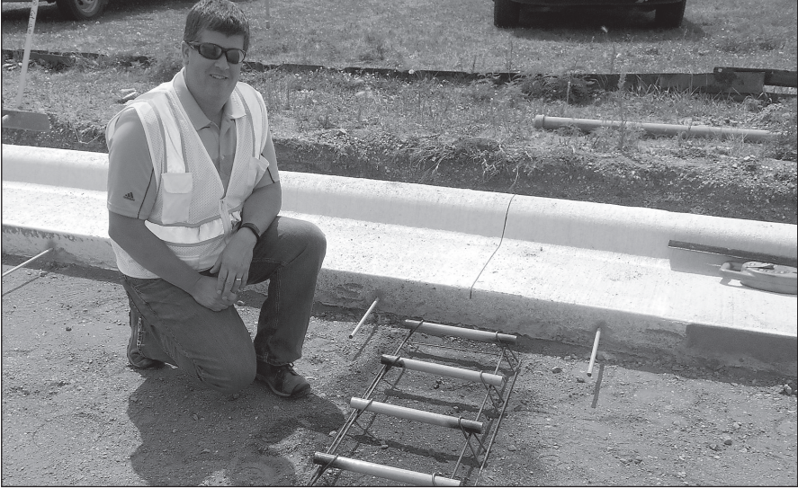
Staff photo by Howard Lestrud Assistant Steele County Highway Department project engineer Stefan Gantert is pictured by concrete dowel baskets, installed in concrete to the east of Highway 218 to help transfer heavy traffic loads. Concrete work has been a priority on the Blooming Prairie Main Street project the past two weeks.
