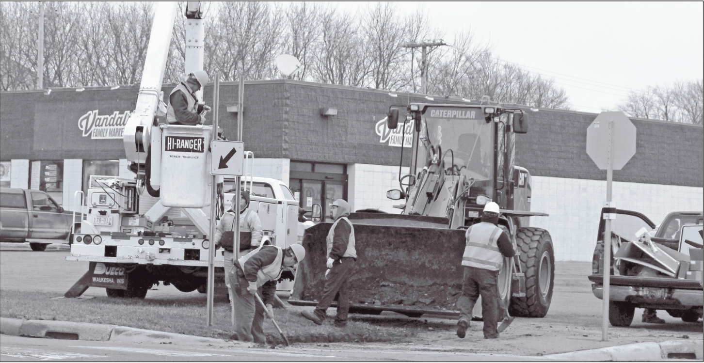
Workers install new LED-lighted crosswalk in Blooming Prairie on Tuesday, Dec. 8. The new crosswalk sign is located at the intersection of Highway Avenue South and Second Street Southeast.
