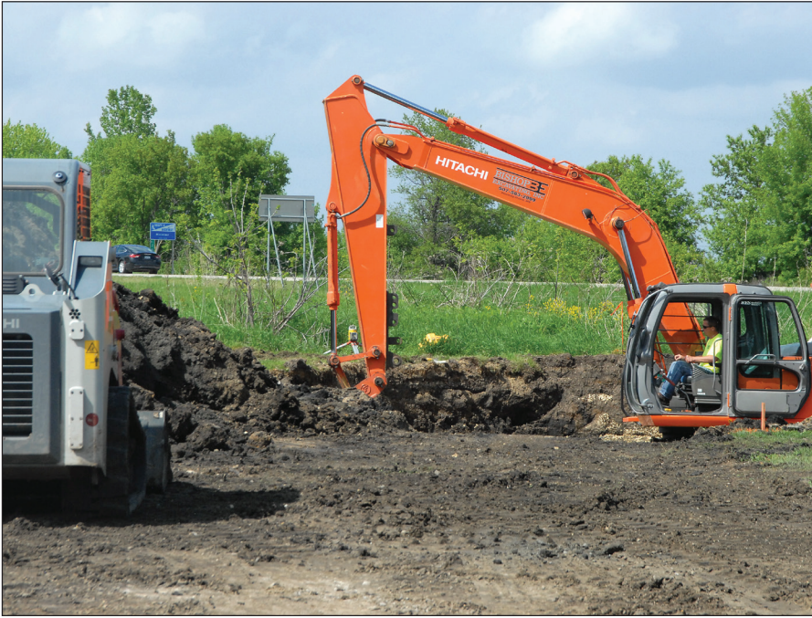
STAFF PHOTO BY HOWARD LESTRUD Groundbreaking for the Blooming Prairie Veterans Memorial is history as of last Saturday. Excavation began in earnest early last week with Bishop Excavating doing the site preparation work. The memorial is expected to be completed by Veteran’s Day.
